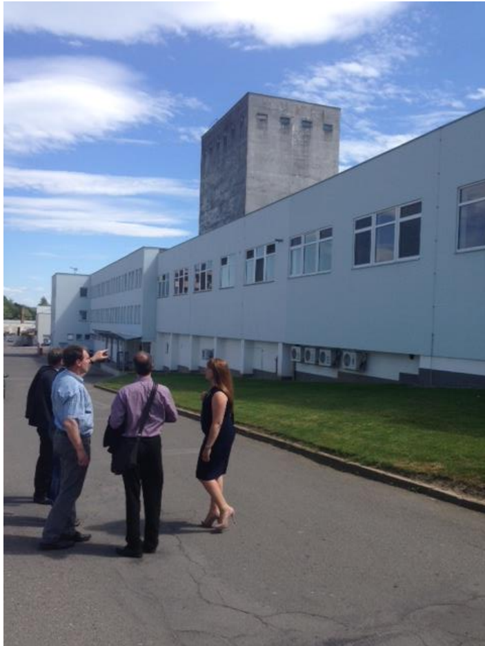
External wall insulation
